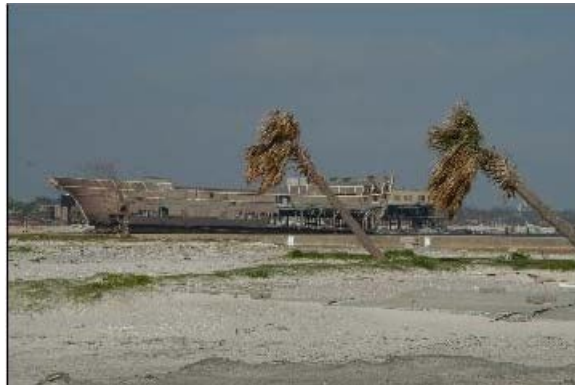
Figure D-3 Strong Wind Effects (Source: FEMA)
