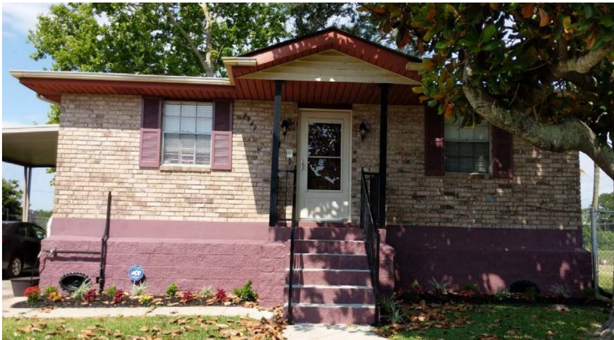
Figure 1- 9 Example Elevated property in Lincoln Manor
