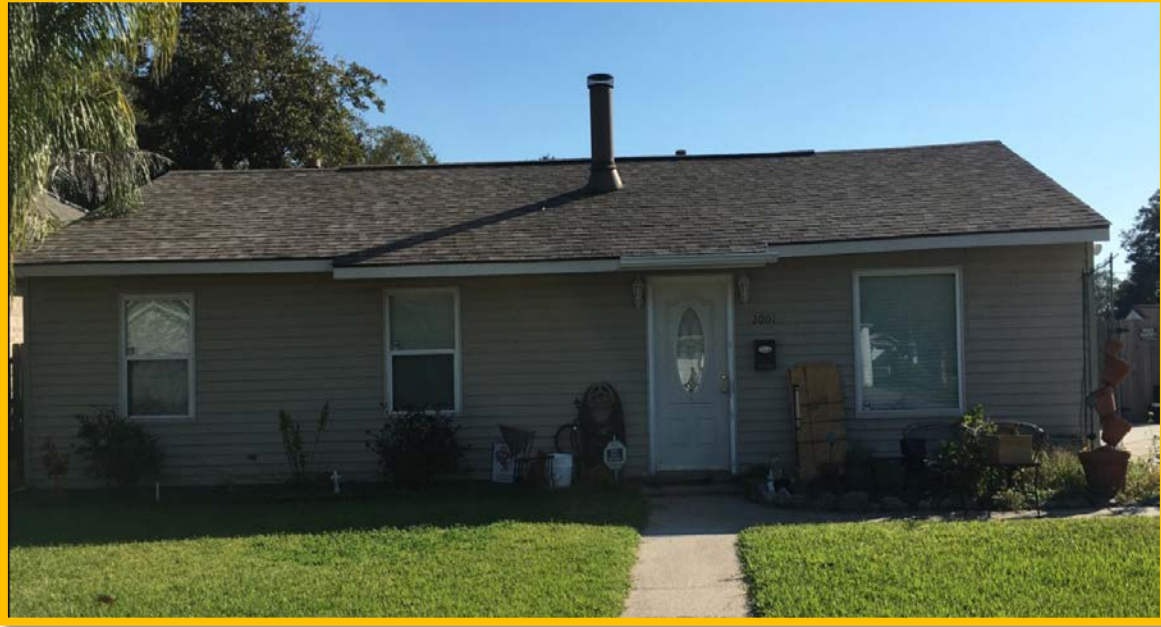
Figure 4- 6 Sample Slab on Grade Structure in Subarea 4
