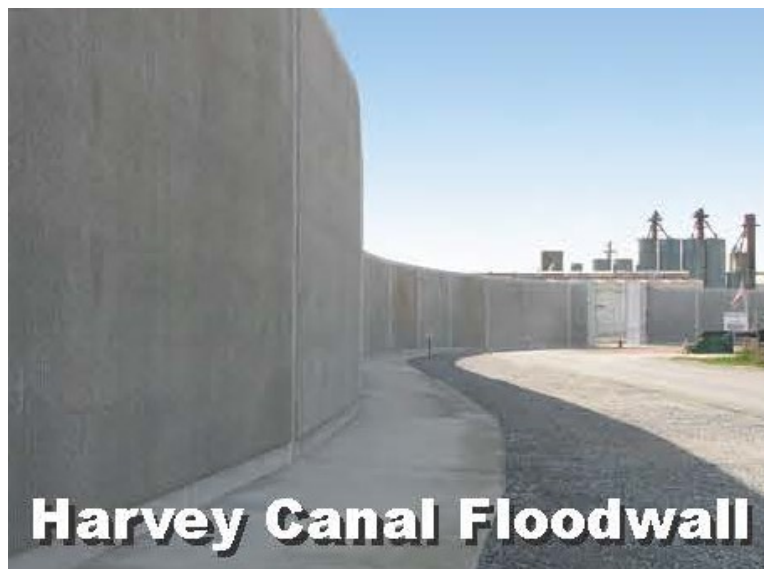
Figure 54 Army Corps of Engineers Harvey Canal Floodwall
