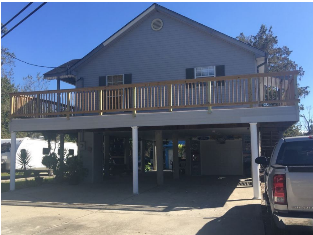
Figure 2-10 Example elevated property in study area
