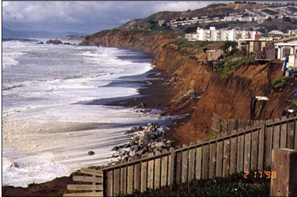
Figure D-5 Coastal Erosion in Pacifica, California During El Niño Year in 1998 (Source: USGS)
