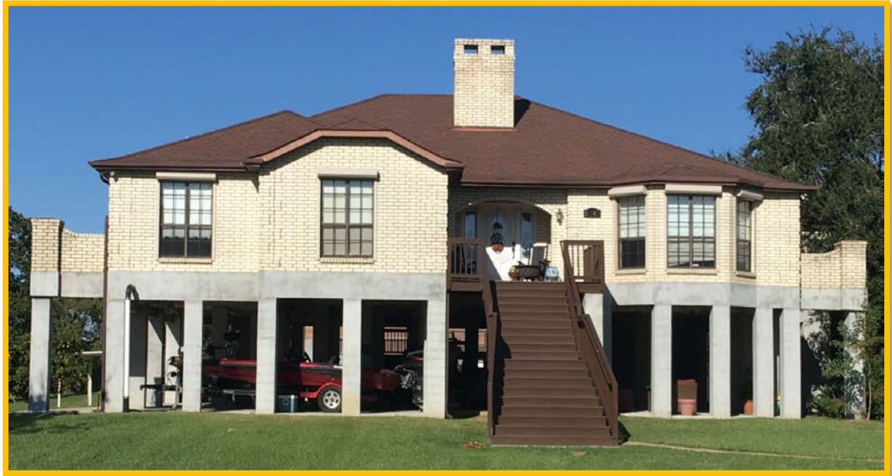
Figure 1- 8 Example of mitigated property in Subarea 1
