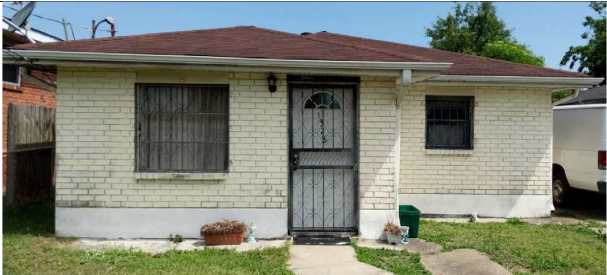
Figure 1- 8 Example Slab on Grade property in Lincoln Manor
